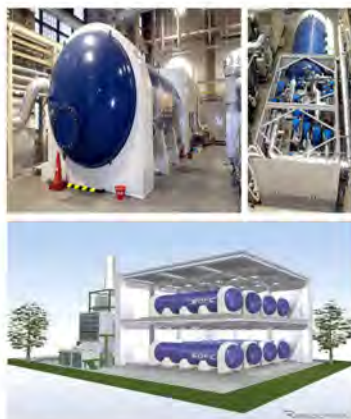
SOFC(50)-GT(35)-ST(15) Triple system
